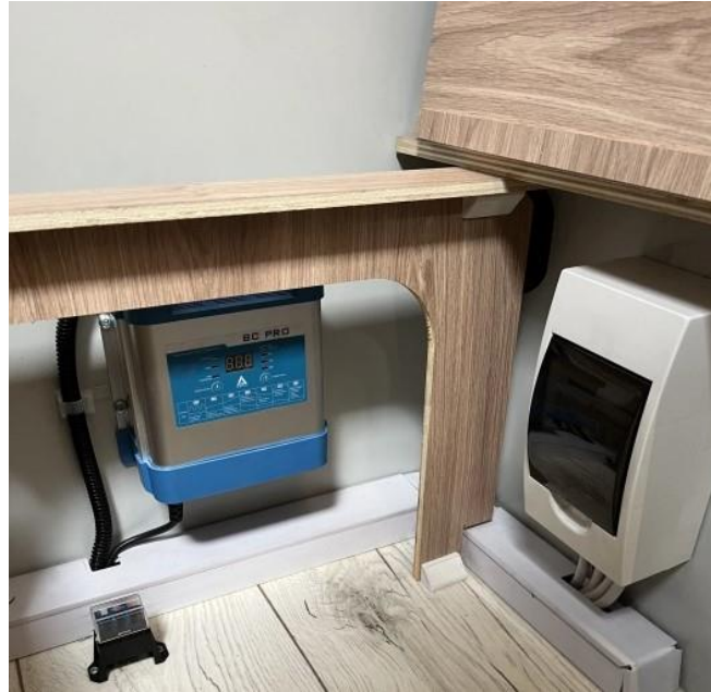
Figure 3. Power supply unit with fuse box
